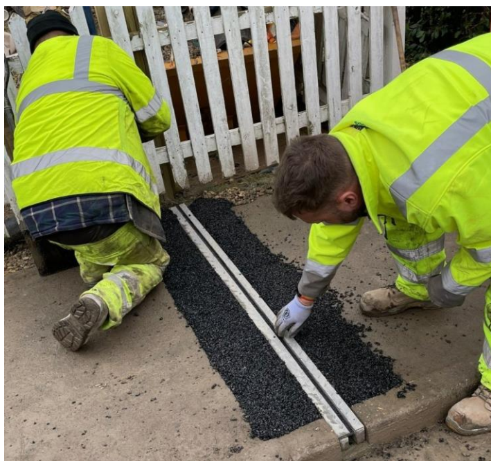
Figure 5 - Buckinghamshire Highways installing in-pavement channel in Wendover.
